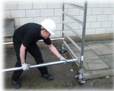
Fit 2 horizontal braces to the vertical member of the frame as low down as possible.
