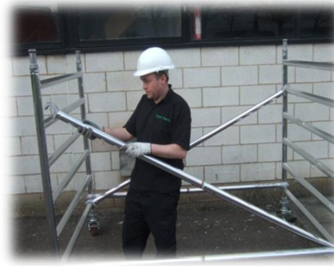
Fit in 2 diagonal braces, starting at the bottom rung – on opposing sides.
