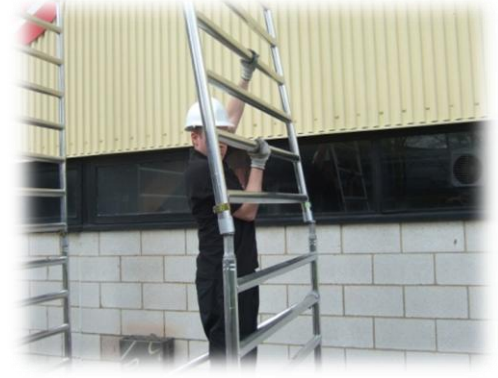
Add 2 frames, after adding any frames always engage the interlock clips
