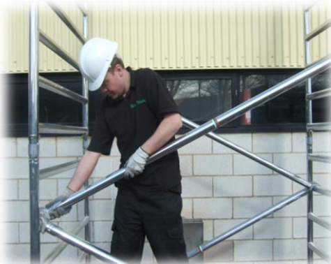
Lock Castors and level the tower, Insert diagonal braces in a regular pattern opposing each other as illustrated.
