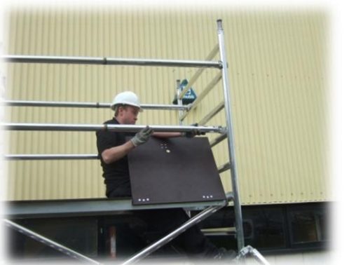
From the sitting position, through the trapdoor (3T Method) Fit horizontal braces as mid rails and guardrails to the vertical member, Hooks facing outwards.
