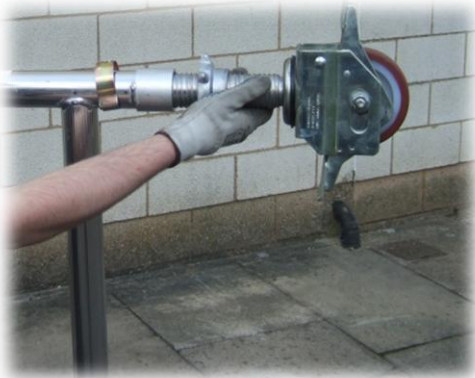
Insert Castors and adjustable legs into frames.
