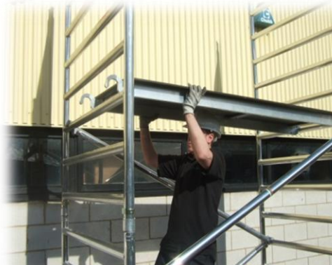
Put platform on the 9 th rung.
