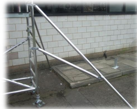
Fit stabilizers at this point
